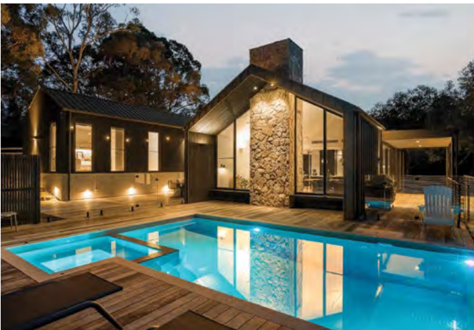
Hopetoun House YSC Architects
