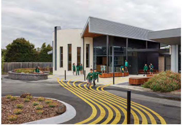
St Clare's Primary School, Thomastown – Harmony Building & New School Entry MUSK Architecture Studio
